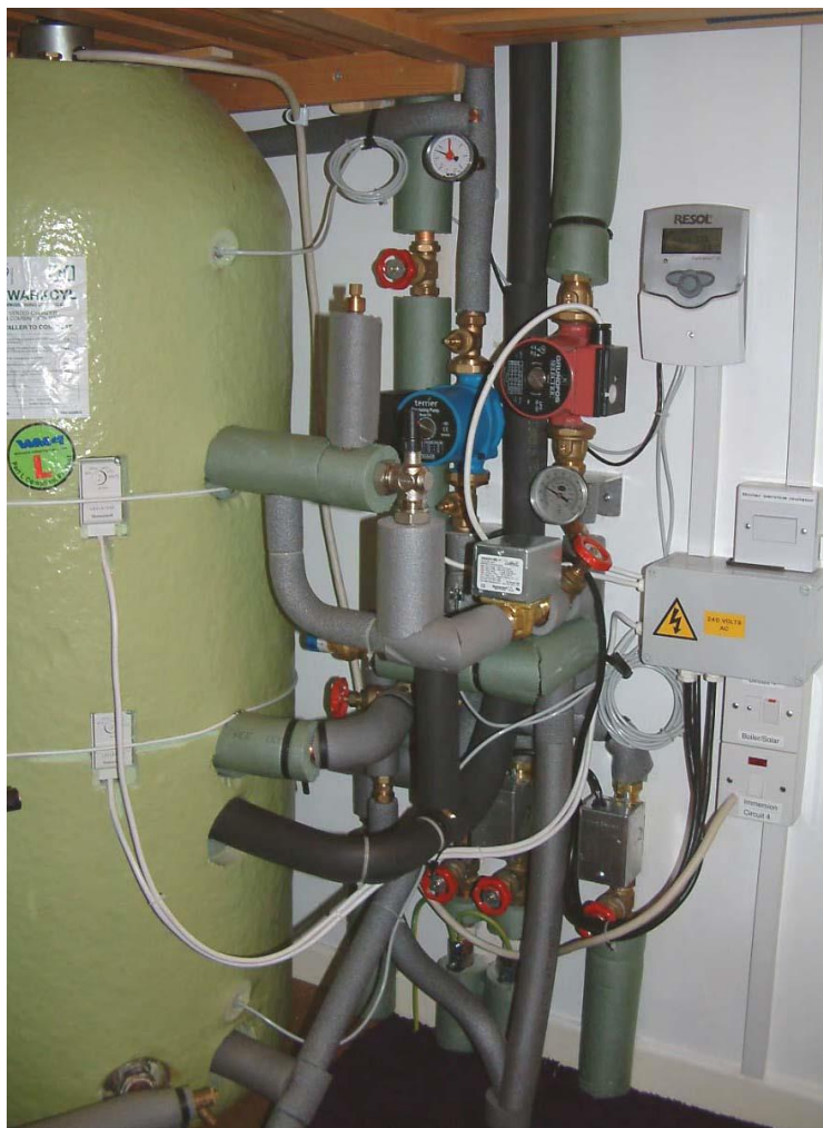
Completed boiler and solar pipework and flow controls
