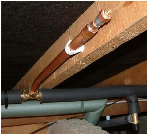
*Flow pipe air vent detail and pressure relief valve*
