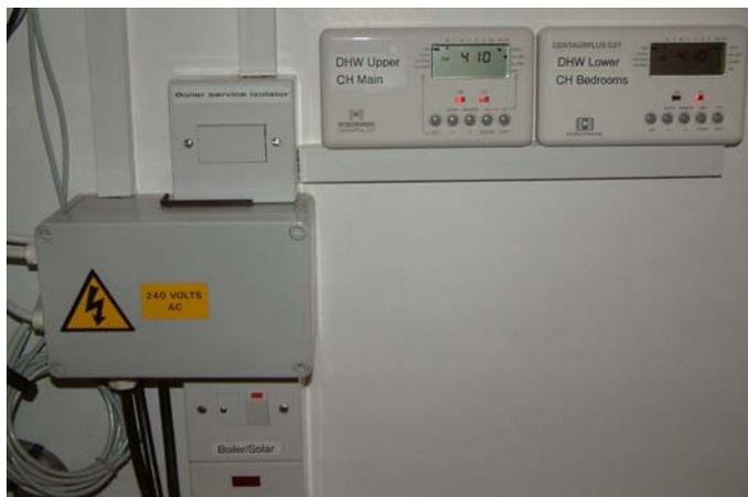
*Twin programmers and electrical control installation*
