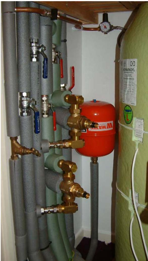
*New valve gear and TMVs – part of solar filling-loop and Pressure Regulating Valve at top*
