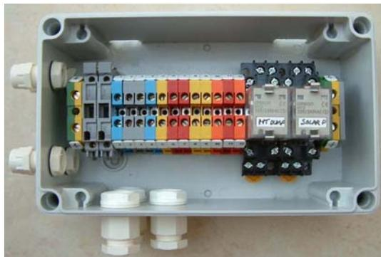
*Main wiring terminal and relay box for combined heating and solar wiring*
