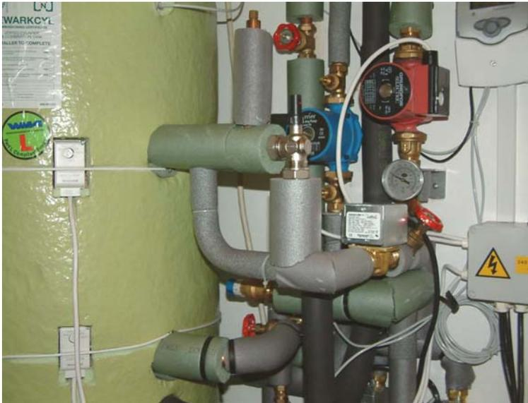
*ADPBV detail on boiler coil – main system ADPBV in background (blue cap)*
